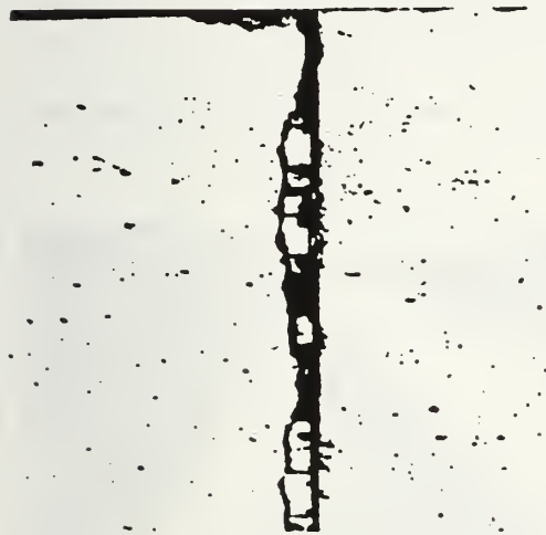
Fig. 3.2.3.9 — Joint spalling
